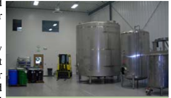
Blending Bay at New Facility
