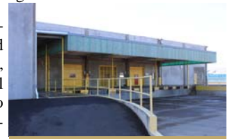
Distribution Warehouse Dock
